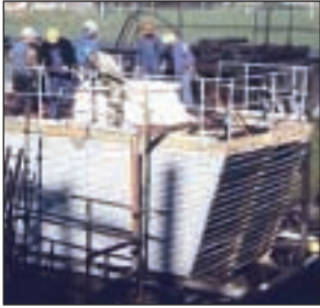
Lakeside's first cooling tower built under license.
