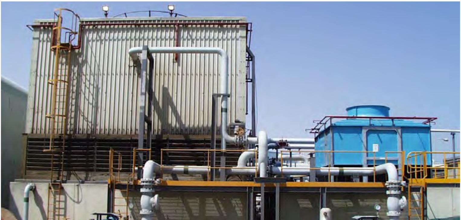
The picture above shows a typical result of our design and manufacturing success. On the left it shows a typical old design cooling tower that is replaced by Lakeside's designed cooling tower that is 1/8th in size and consumes a proportional reduction in energy. This installation provides the necessary cooling for Dubai Aluminium's die casting plant.
